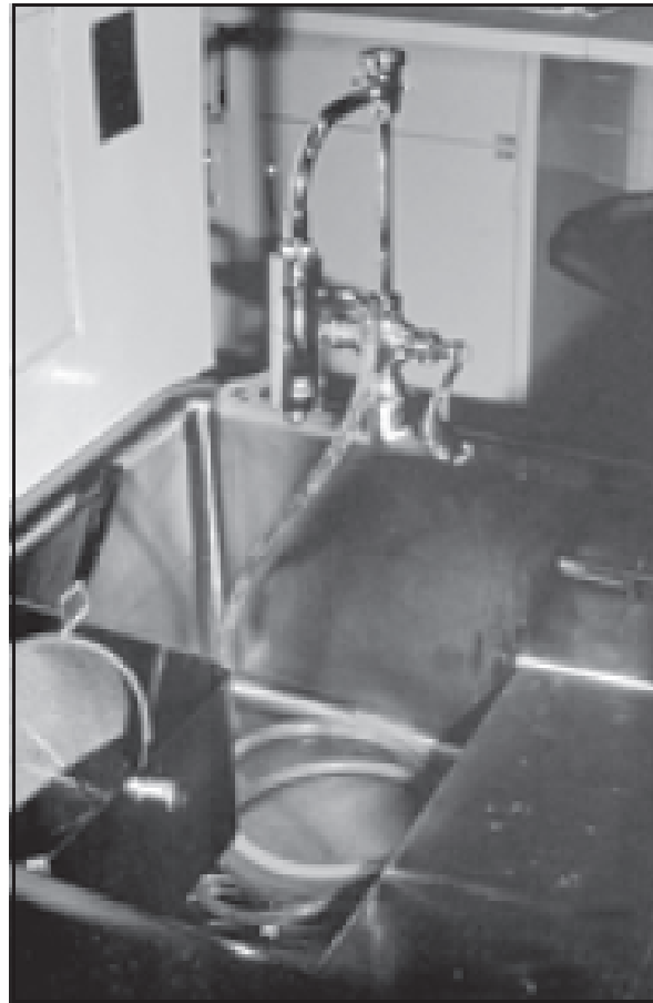
FIGURE 17. Atmospheric vacuum breaker in plumbing supply system.
